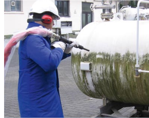
Surface preparation before tank restoration
